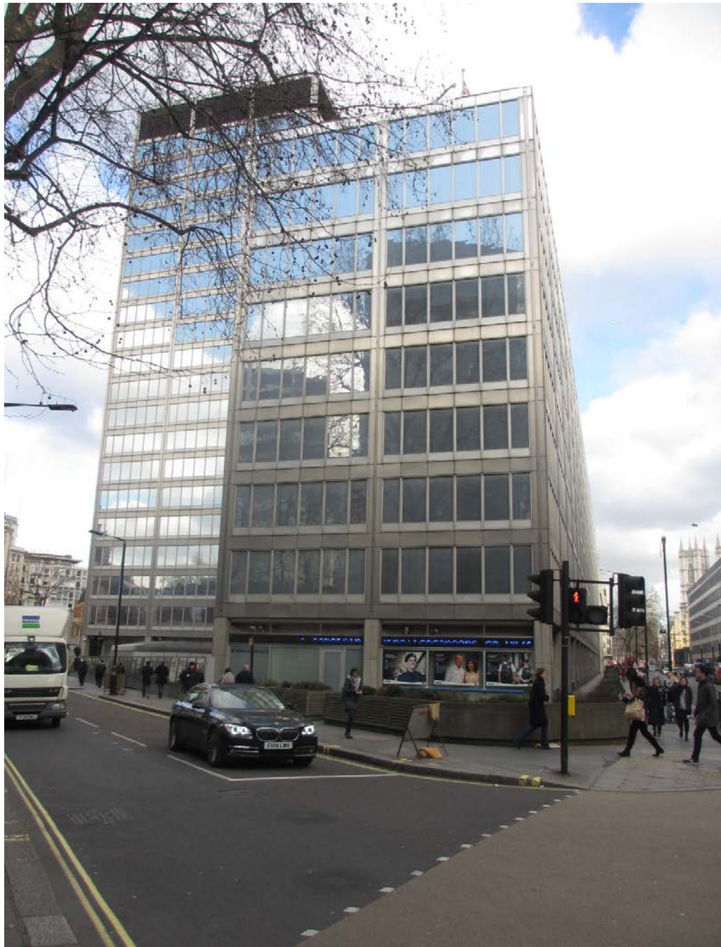
8 – 10 Broadway, New Scotland Yard (view from Victoria Street at corner of Broadway (prior to works))
